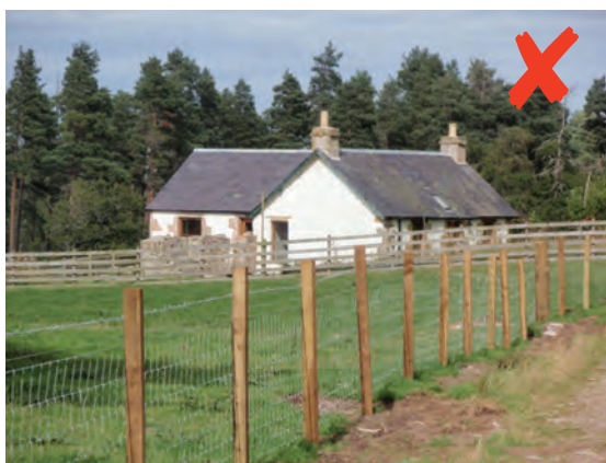
Newly formed post and wire fencing
