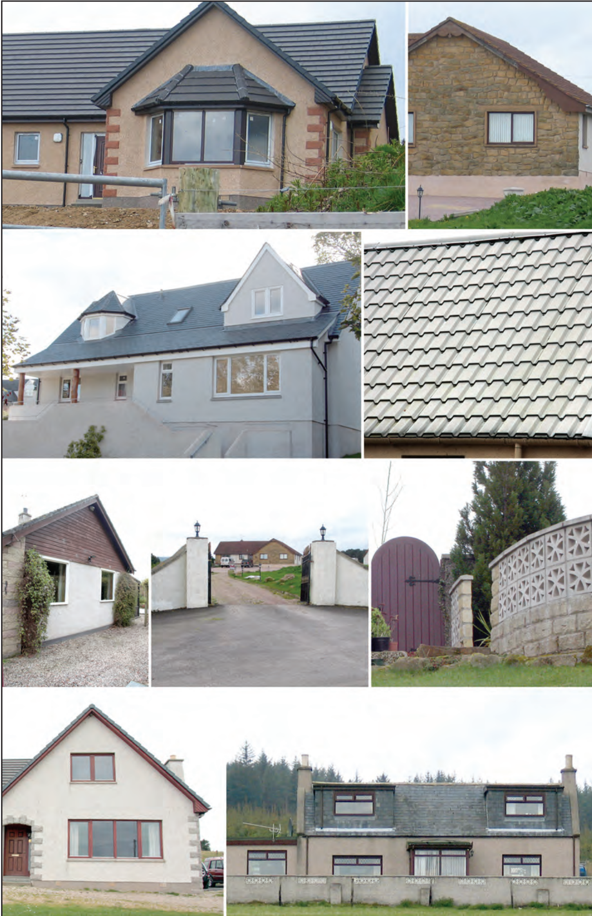
Inappropriate materials and detailing for the rural environment
