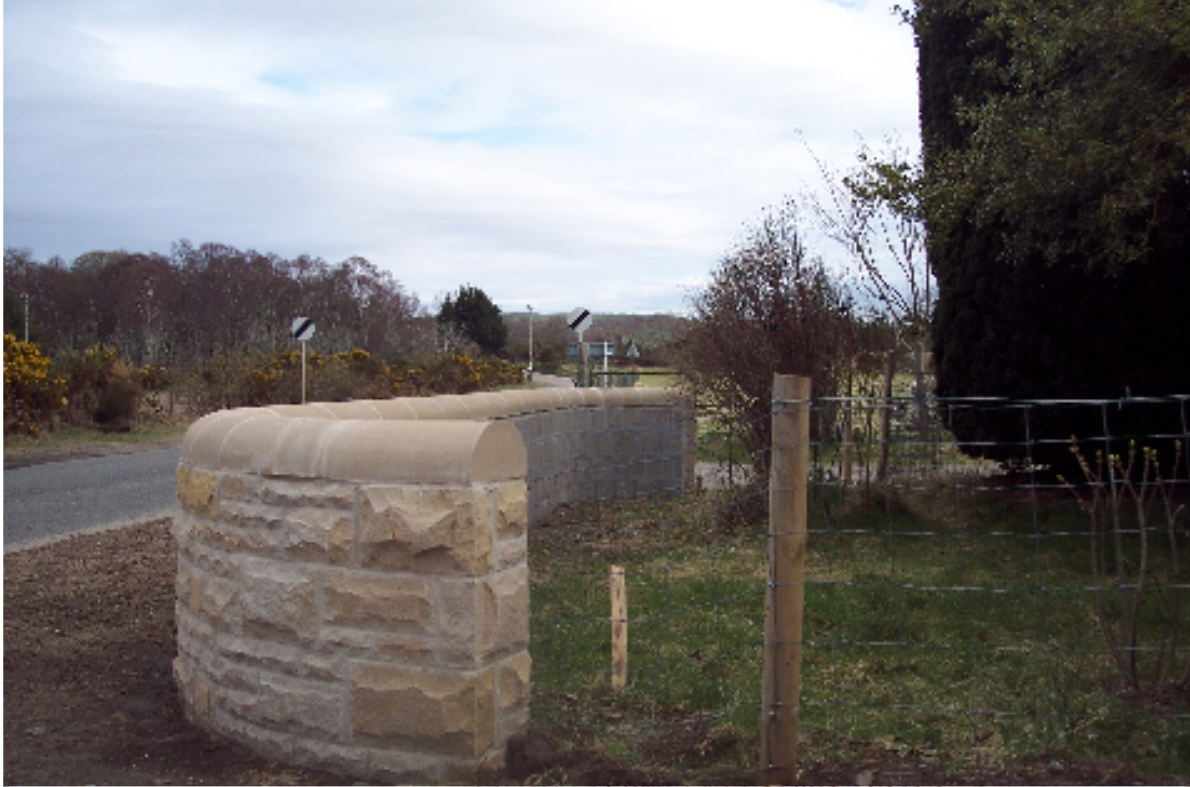
A – Photograph taken at driver’s eye level from an ‘x’ distance of 4.5m, facing South East
