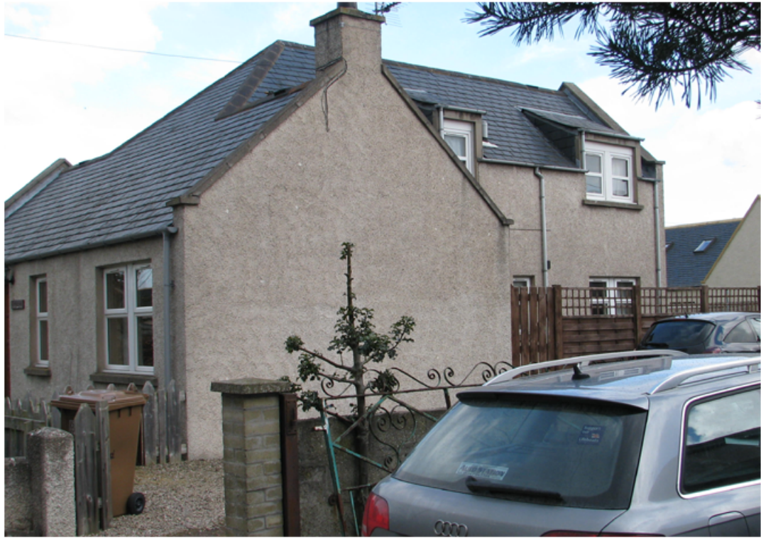
Roof joint involving different ridge heights and wallheads at Grianan (next door to Southview)
