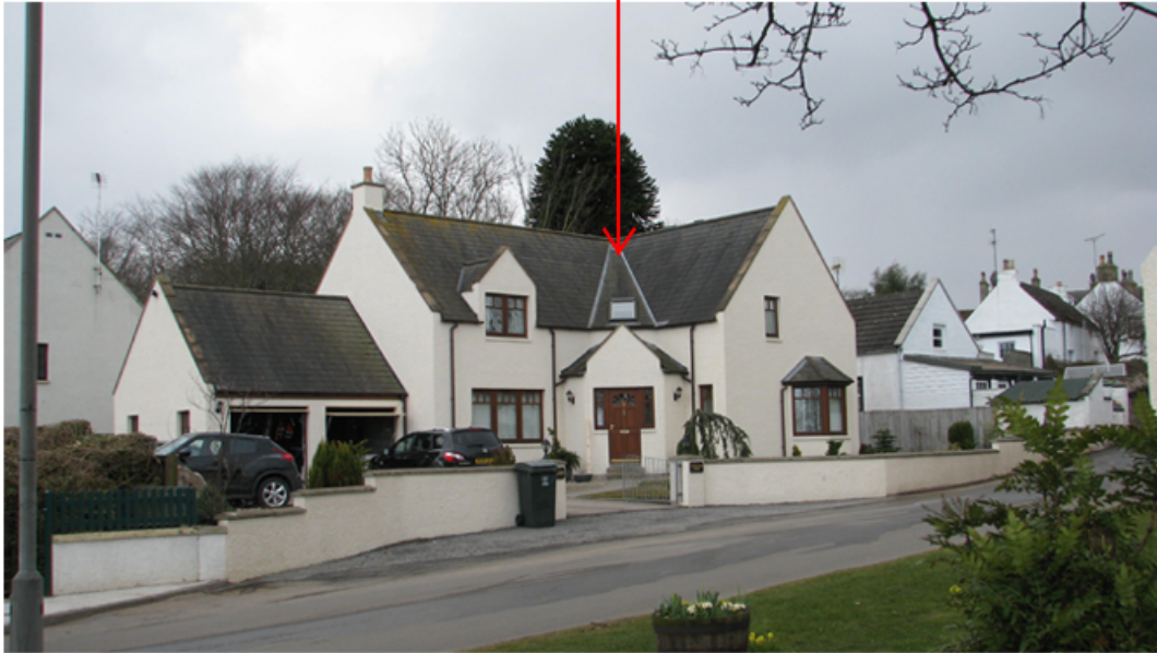
Recently approved unusual roof joint using traditional materials
