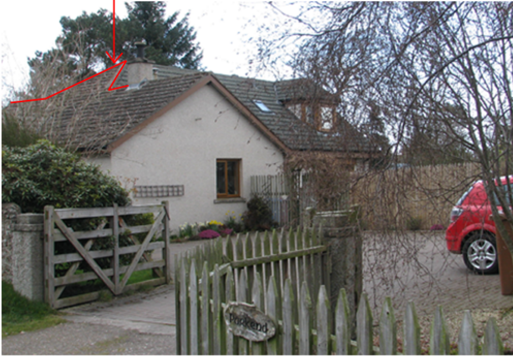
Approved joint of roofs and ridges of differing heights at Parkend similar to that proposed at Southview
