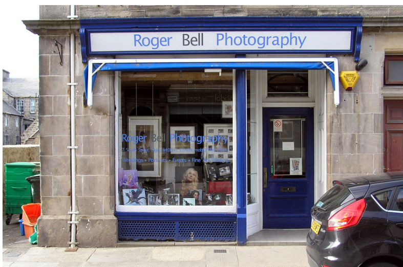
This attractive cast iron shopfront on South Street, although well maintained, suffers from rust damage to the decorative cast iron ventilators within the stall riser for which a small grants scheme might provide financial assistance for what might be an expensive element to repair or replace
