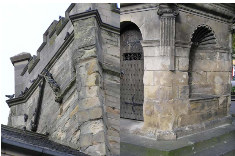
Advanced stone decay: the tower of the former UP Church on Moss Street, suffering from delamination and contour scaling, and with damage evident from plastic repairs having been carried out in cement; the Muckle Cross (right) has suffered from a complete loss of architectural detail in the lower parts of the monument
