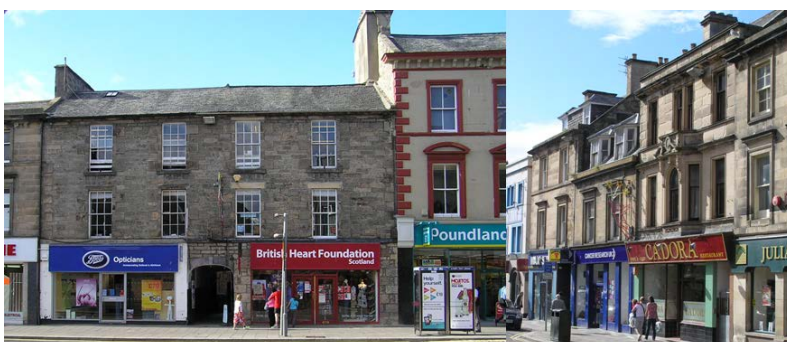
Shops and tenements, of which the earliest is dated 1811, with problems of decay and high level maintenance; as a group the buildings make a strong contribution to the historic townscape and are suggested as a single priority project
