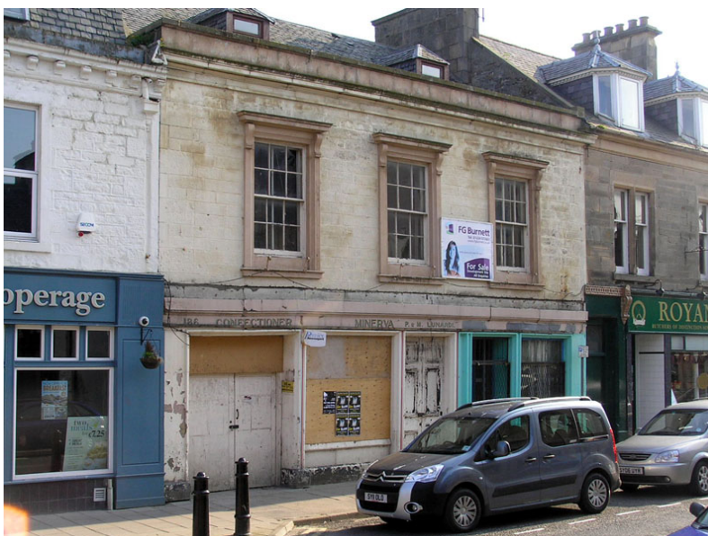
A prominent Category B listed Building at Risk at 186-188 High Street
