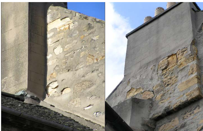
The incidence of decaying soft sandstone made worse by the application of dense cement renders and mortar is common throughout the conservation area
