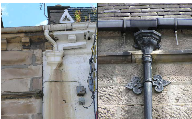
Problems with decorative cast iron rainwater goods – loss of original patterns and replacement in modern profiles and materials
