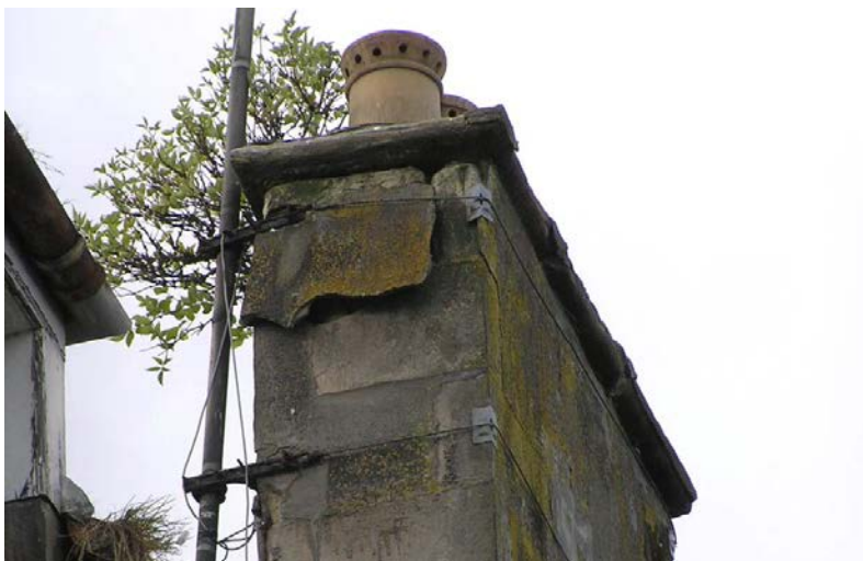
Masonry in a dangerous condition, at risk of falling and causing injury or damage to persons or property
