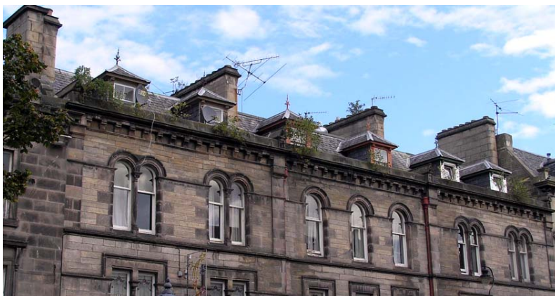
Appreciation of the skyline of a fine late nineteenth century buildings is marred by trees growing out of gutters and open joints in masonry at high level
