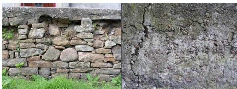
Rarities in the conservation area: a 'rig' wall and a boundary wall of rubble stonework bound with clay mortar, and of mass unreinforced concrete
