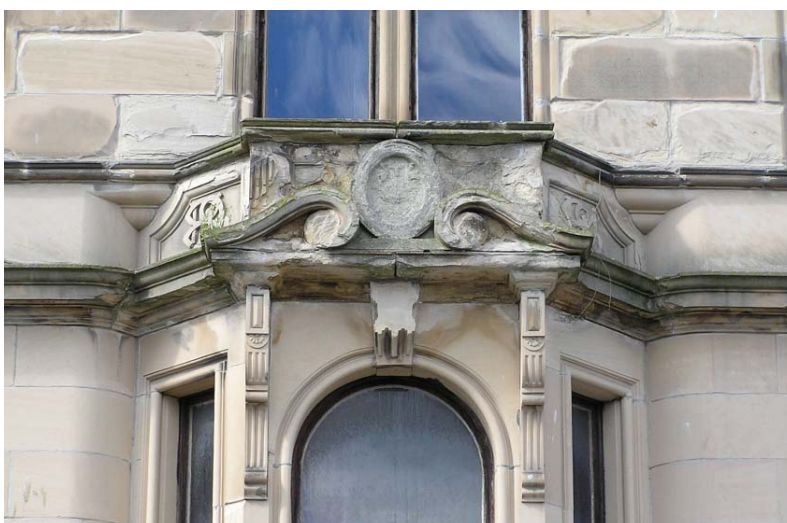
Carved stonework detail to a projecting bay window obliterated from stone decay; weathering back of the face of the stone can be seen around the joints in the ashlar masonry
