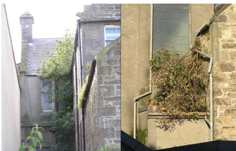
Problems of vegetation growth from lack of maintenance; the tree growing out of the wallhead on the right image has brought down the rainwater pipe
