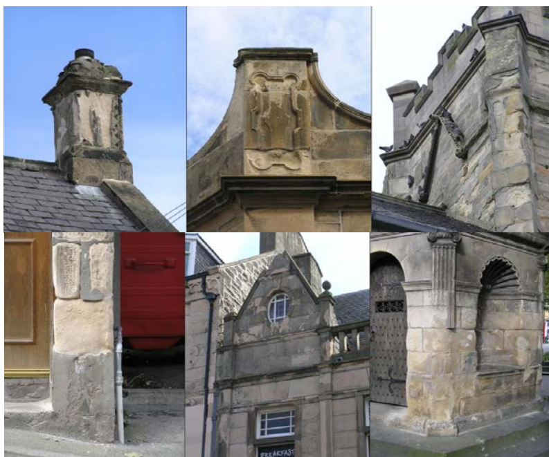
Examples of masonry decay, which in some instances has resulted in the loss of carved architectural detail
