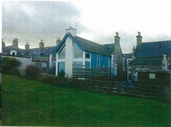
Picture 2. Neighbouring extension.
