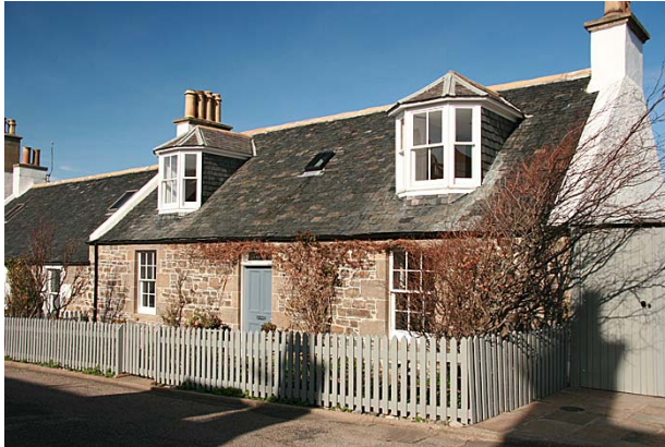
Existing house at 17 Lower Blantyre St as renovated by applicant
