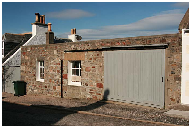
Existing flat roofed bothy
