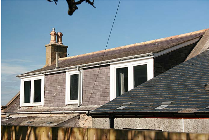
Existing dormer at rear of 1 Campbell St
