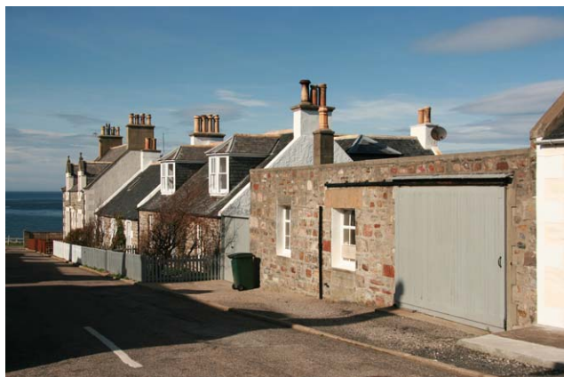
Existing flat roofed bothy and adjacent houses
