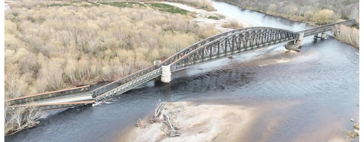
The failed spans in the River Spey
