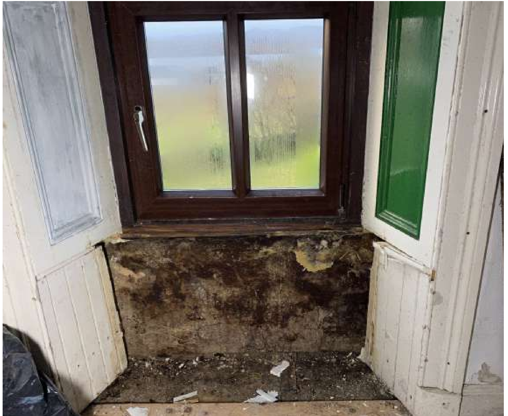
Example of inappropriate modern interventions which lead to deterioration of traditional fabric.
