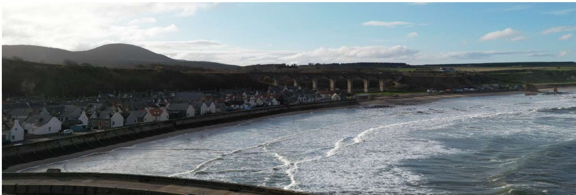
Portknockie Seatown and Viaduct Aerial Image
