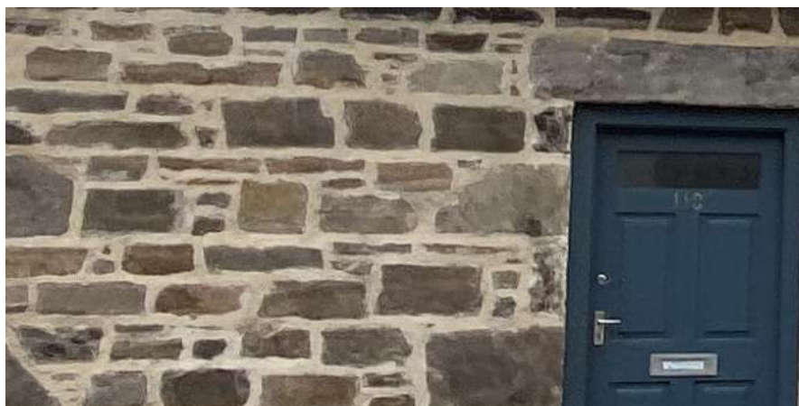
Lime pointing to the traditional walls with a timber door.
