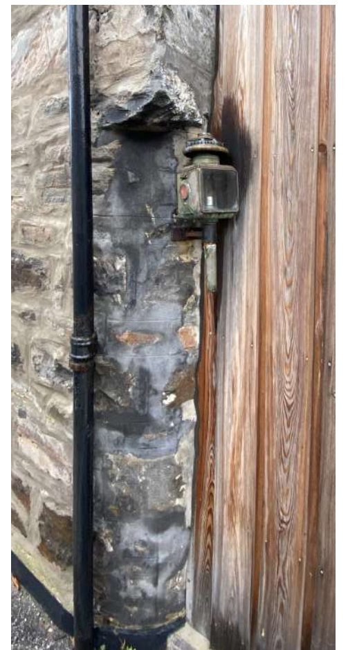
Heritage fitments are evident in Cullen
