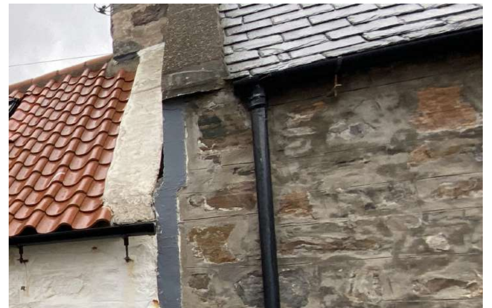
Traditional cast iron rainwater goods are evident in Seatown.
