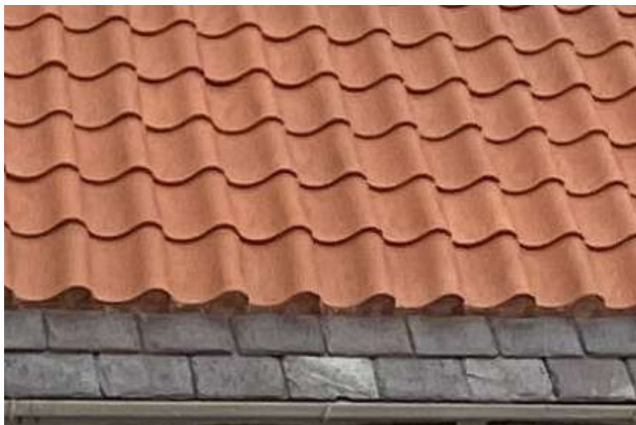
Pantiles with two slate courses to allow for rainwater disposal.
