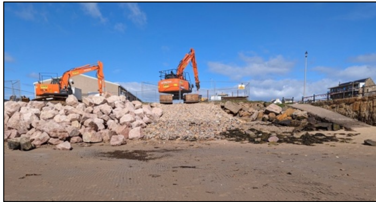
Rock armour being replaced in summer 2023, and the tarmac ramp.
