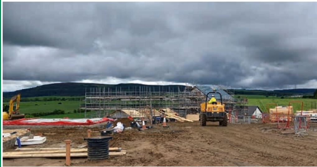
Construction work underway at phase 2, Banff Road in Keith
