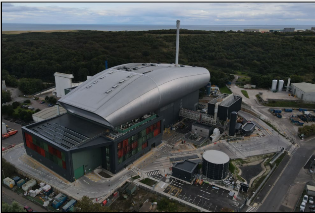
Energy from Waste facility fully operational
