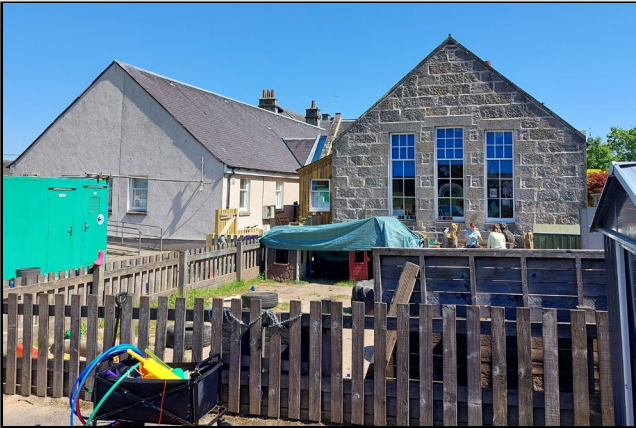
Aberlour Nursery refurbished
