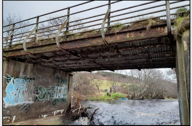
UK Government awards £1.5m for Cloddach bridge repairs
