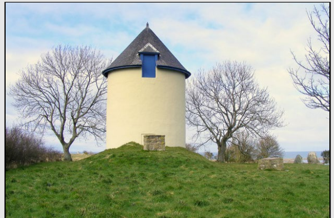
CAT for Garmouth Water Tower
