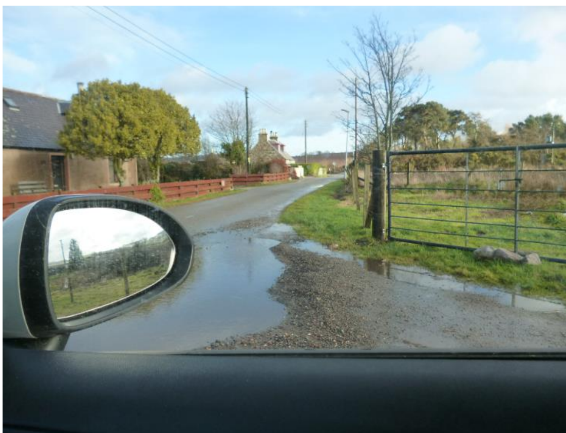
Drivers eye view to east from exiting vehicle – note the significant improvement afforded by the set back fence
