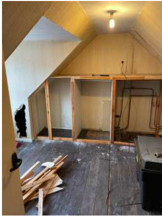
057 East bedroom - 1st floor removing tank housing to gable wall
