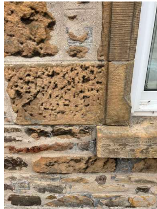
008 front window jamb/lintel stone detail
