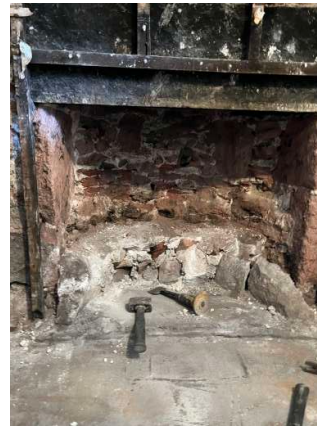
043 west living room fireplace opening removing stone fill during 2022
