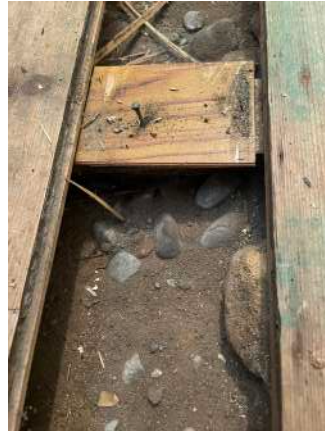
067 void under kitchen floor
