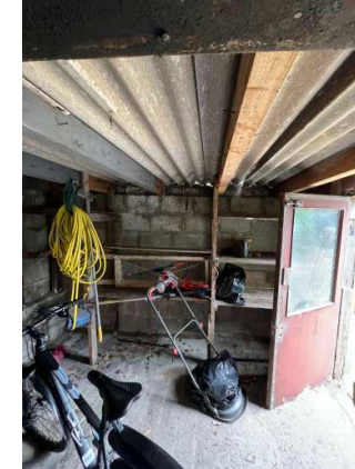
029 north elevation inside garden store
