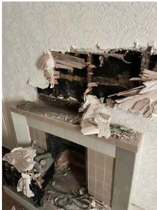
041 west living room fireplace repairs during 2021
