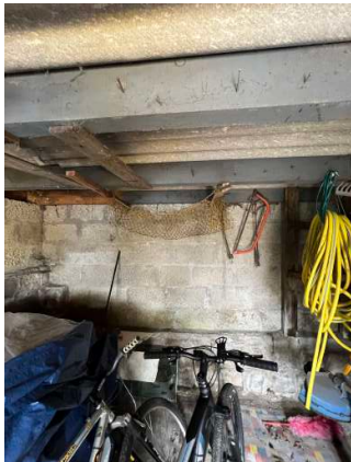
026 west elevation inside garden store
