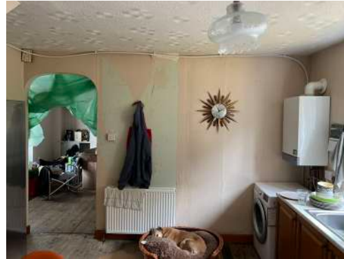
052 kitchen view east
