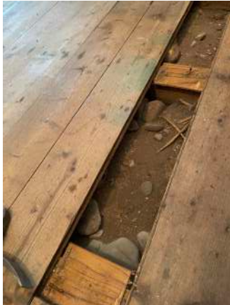
066 void under kitchen floor
