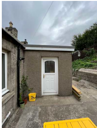
017 west elevation bathroom
