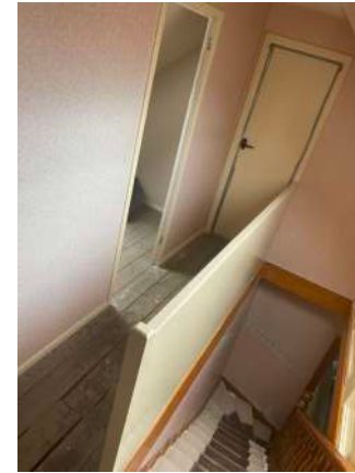
060 first floor landing/passage/stair 2021
