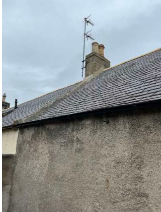
021 south elevation - west chimney
