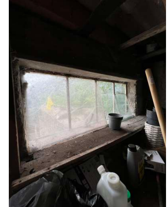
025 east garden store window inside - steel
