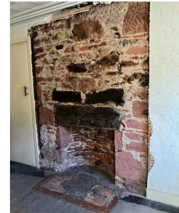
045 west living room fireplace reopened
