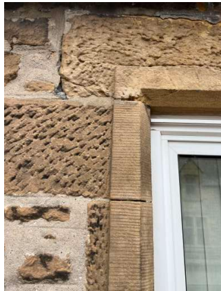
007 front window jamb/lintel stone detail
