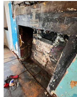
039 east living room fireplace repairs during 2021
