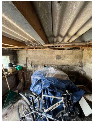
027 south elevation inside garden store
