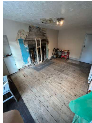
038 east living room fireplace repairs during 2021
