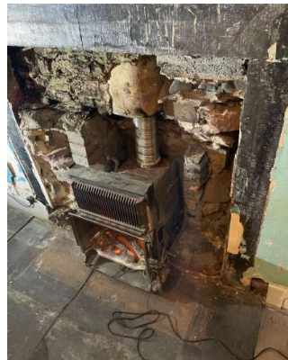
037 east living room original gas fire back boiler during removal 2021
