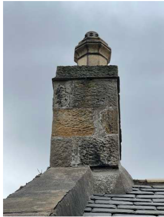
012 east gable chimney
