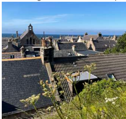
Portgordon varied roofscape
