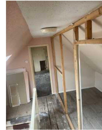
061 first floor landing/passage/stair removing partition wall 2021
