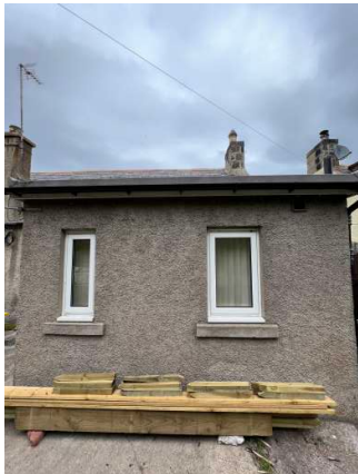
016 south elevation bathroom
