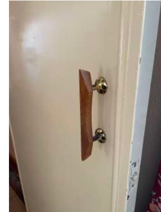
069 ground floor internal door pull handles
