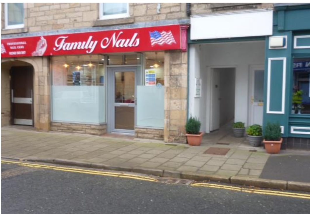
View from High Street of existing narrow private lane
