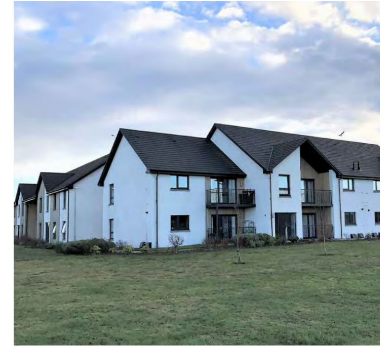
Projecting and recessed balconies (Glassgreen South)
