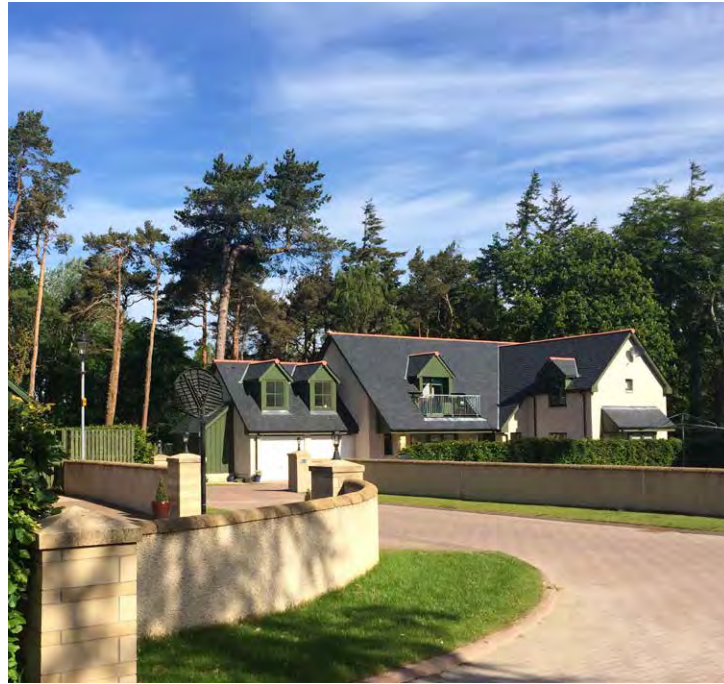
Cladding to match the tree lined backdrop (Dunkinty)
