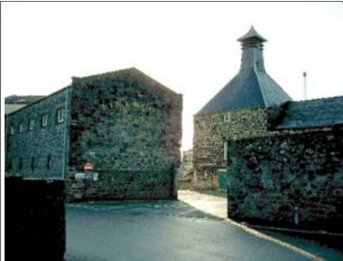
Figure 2 Linkwood Bonded Warehouse, showing Doig Ventilator
