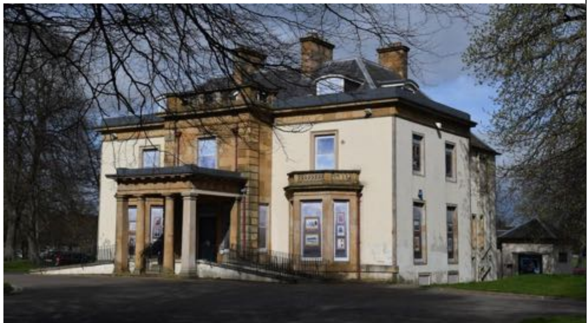
Figure 26 Grant Lodge, Cooper Park
