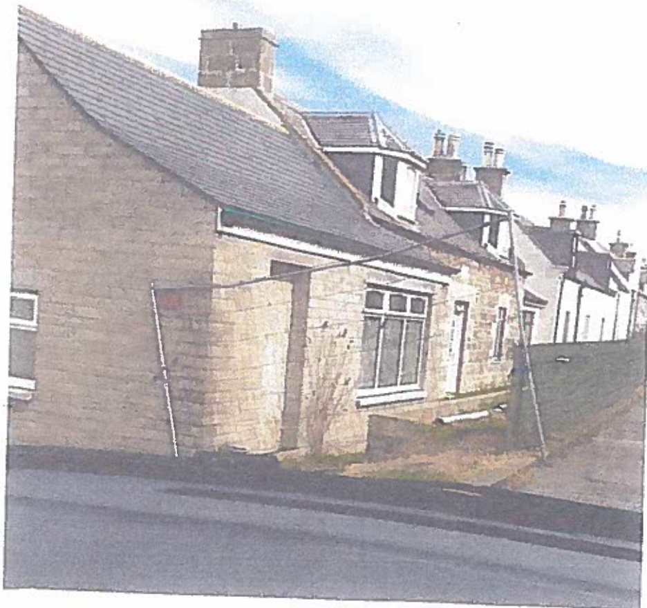
EXTENSION TO TOP WEST SIDE OF HARBOUR ROAD UNDER CONSTRUCTION,
