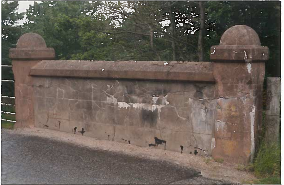
DAMAGED PILASTER
