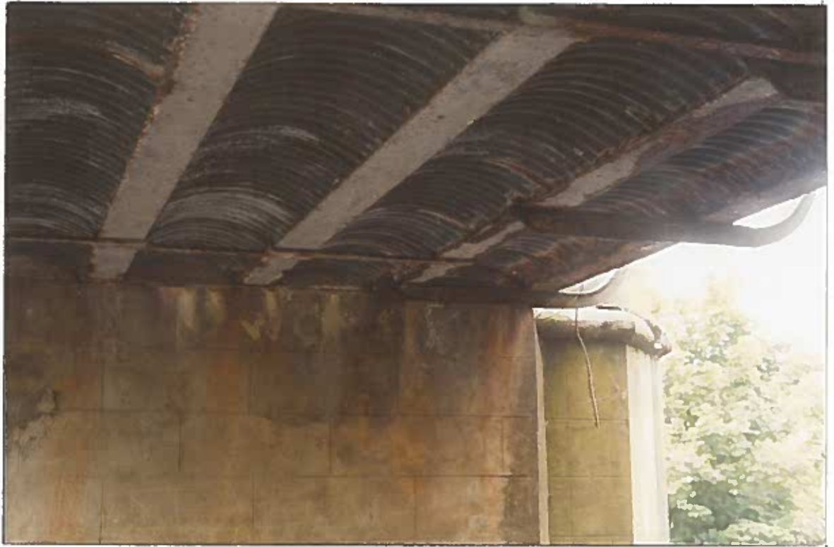
JACK ARCH SOFFIT
