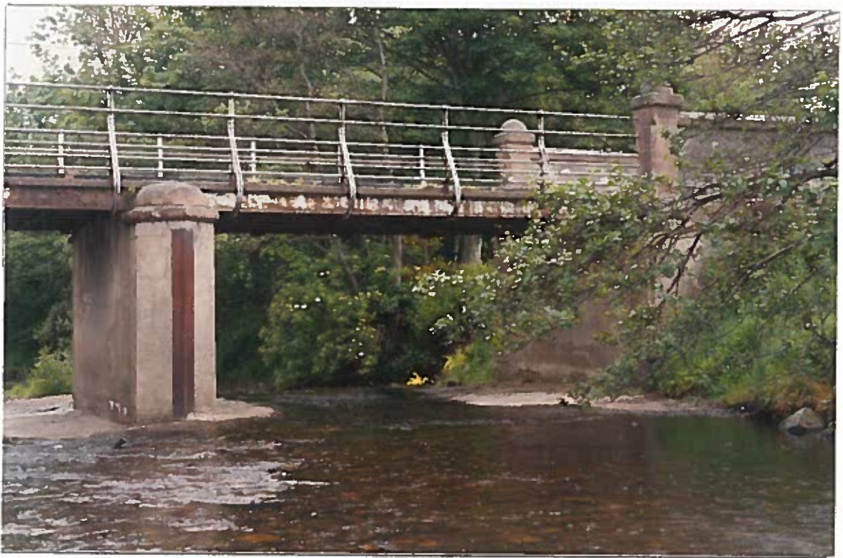
BRIDGE PIERS AND DECK
