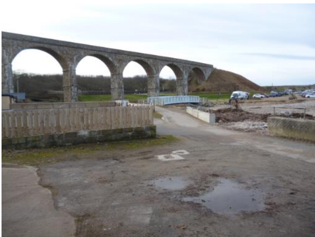
View from existing store frontage onto Core path
