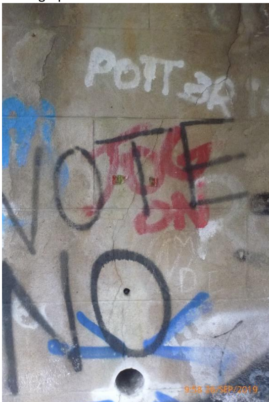
Photograph 19: Vertical crack on West Abutment, with broken crack gauge (0.8mm)
