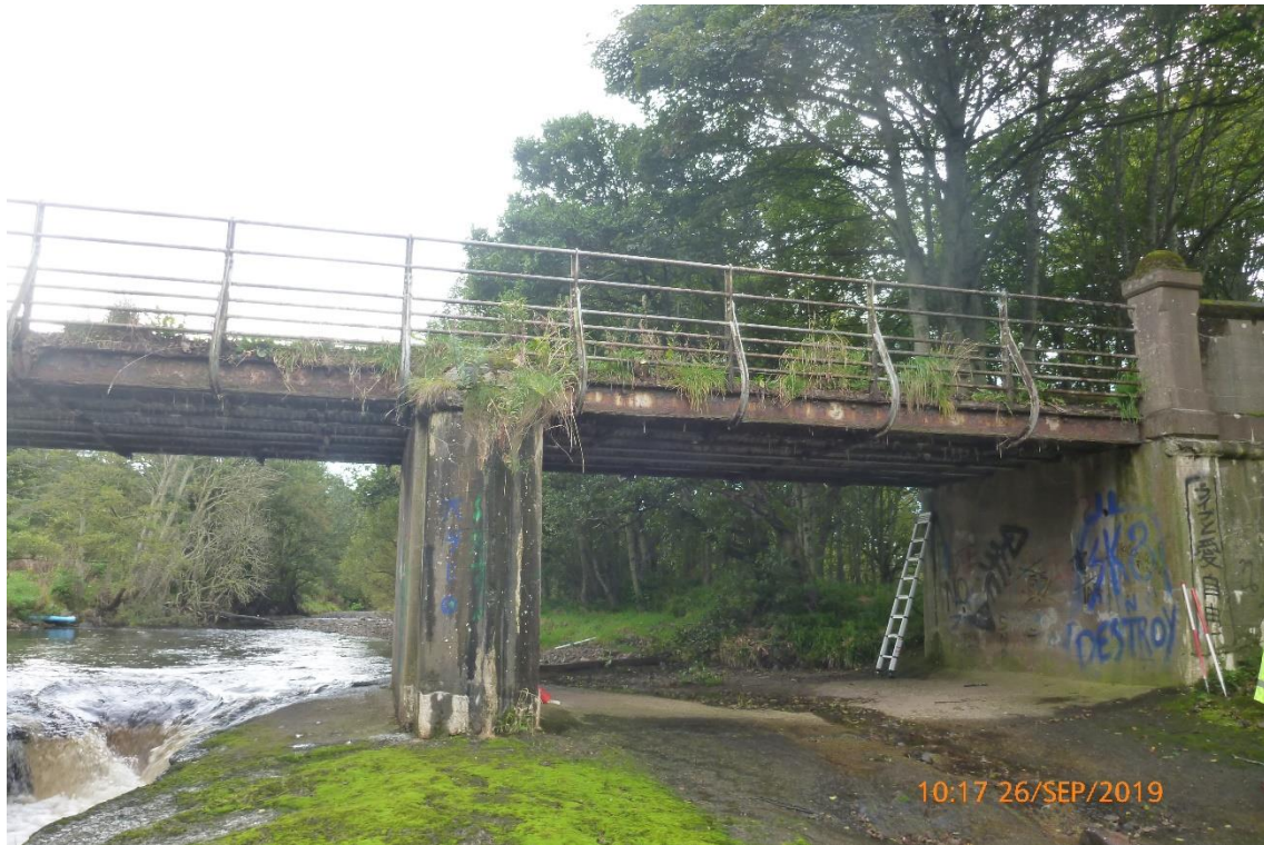
Photograph 1: General view looking South (Span 1)
