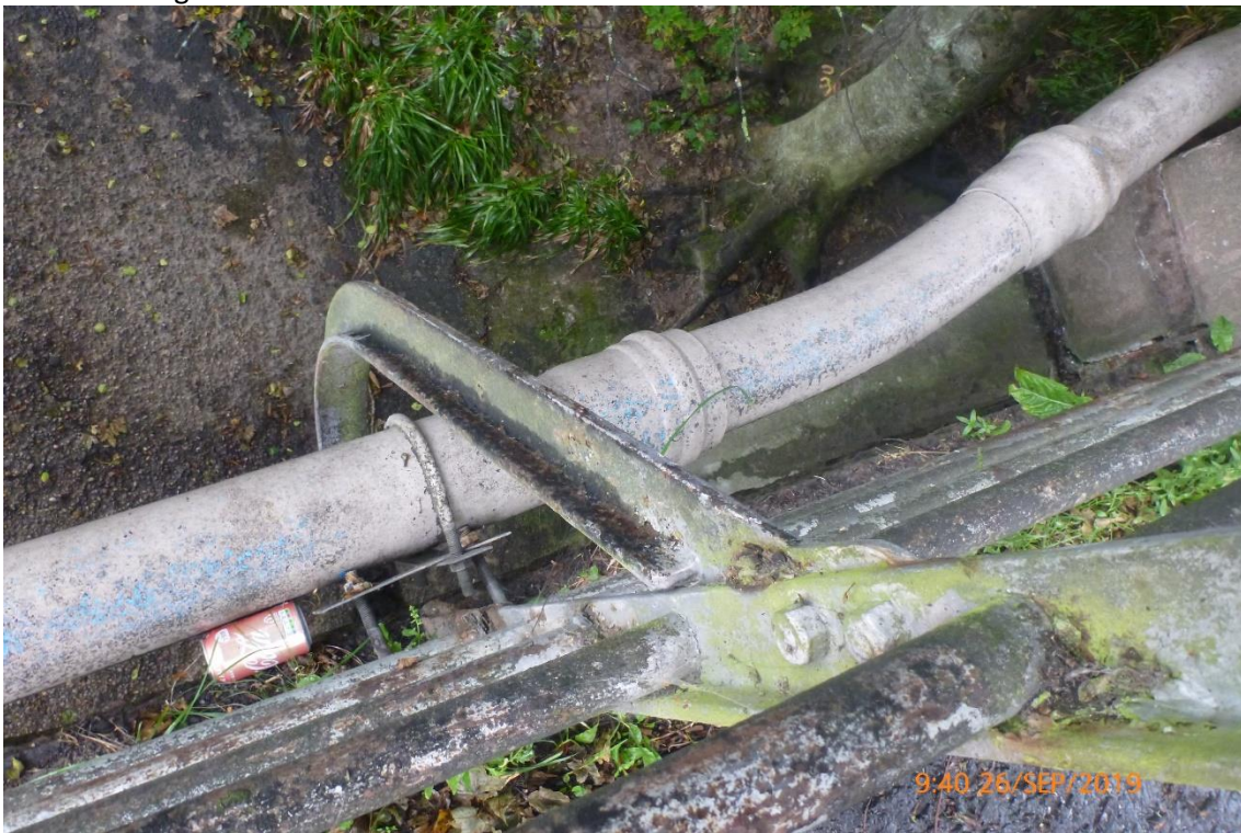
Photograph 32: Pipeline connection to bridge parapets.
