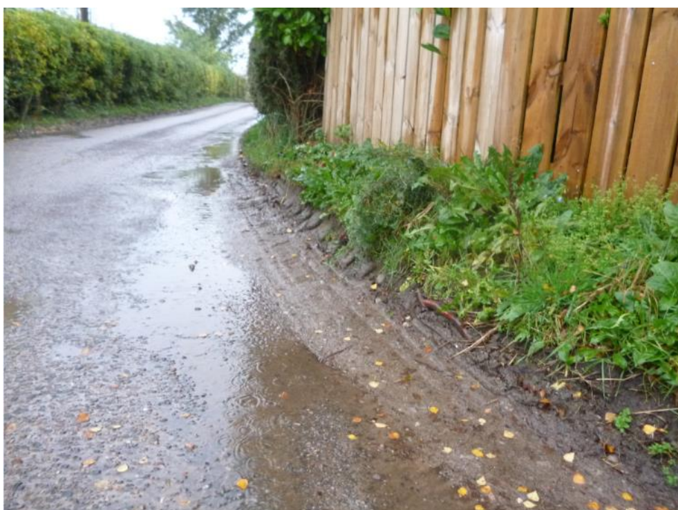
PHOTO SHOWING NARROW VERGE AND EVIDENCE OF VEHICLE VERGE OVERRUNING
