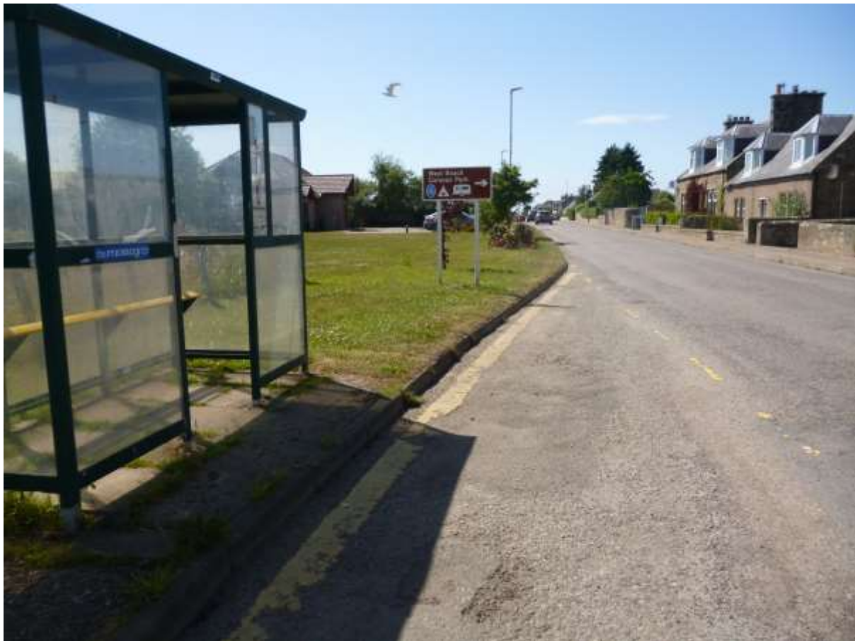
Photograph T004 – Showing view west from westbound bus stop located to the east of the development and missing footway.
