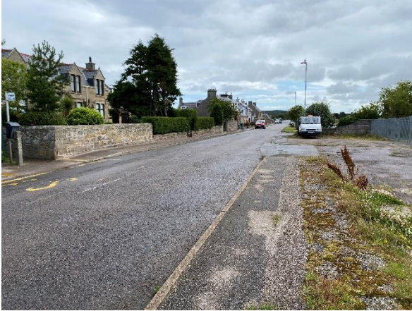
Figure 4: View of facilities on Forsyth Street looking east
