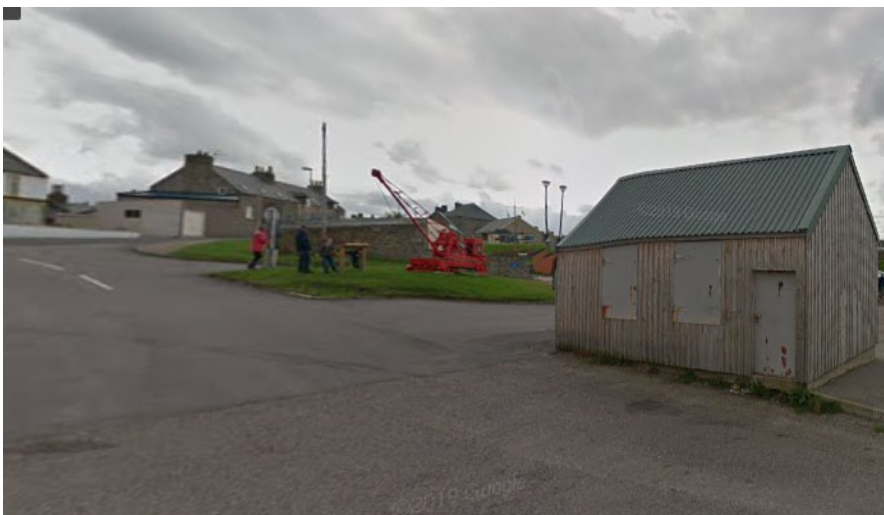
Timber building (off of Harbour Street)
