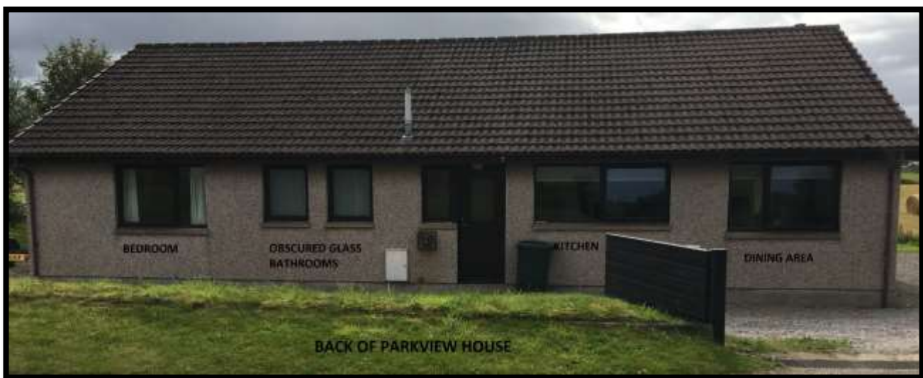
Photo 23: Rear Elevation of Parkview showing windows (and associated use of rooms) © Proctor
