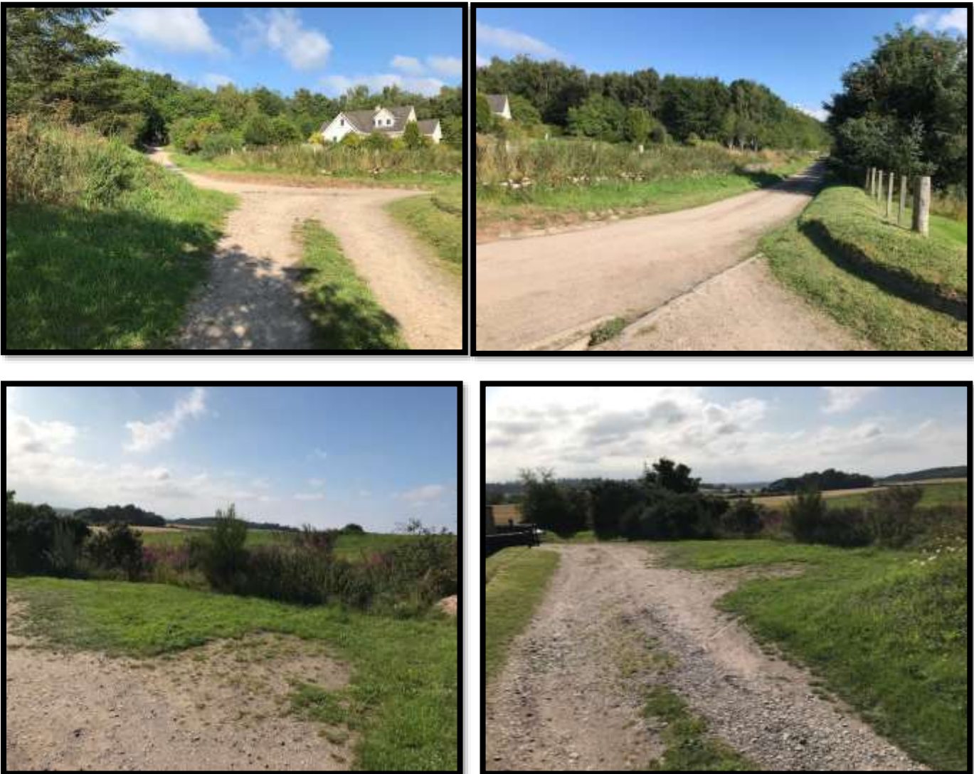
Photos 14, 15, 16 & 17: Roads details: Junction of existing track onto U102E, the track and the junction with the proposed driveway
