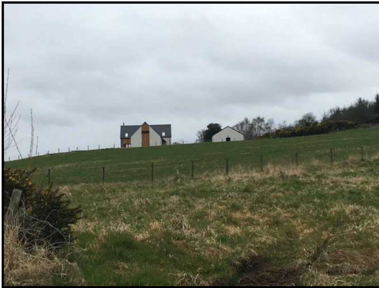
Photograph 15: New Build at Blervie (showing prominence and lack of enclosure or containment)
