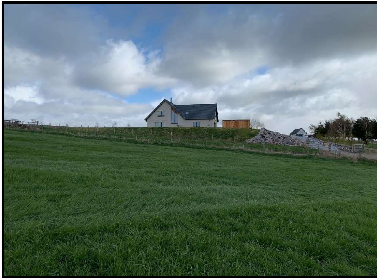
Photograph 12: New Build at Blervie (showing prominence on raised land with no landscape enclosure or containment)
