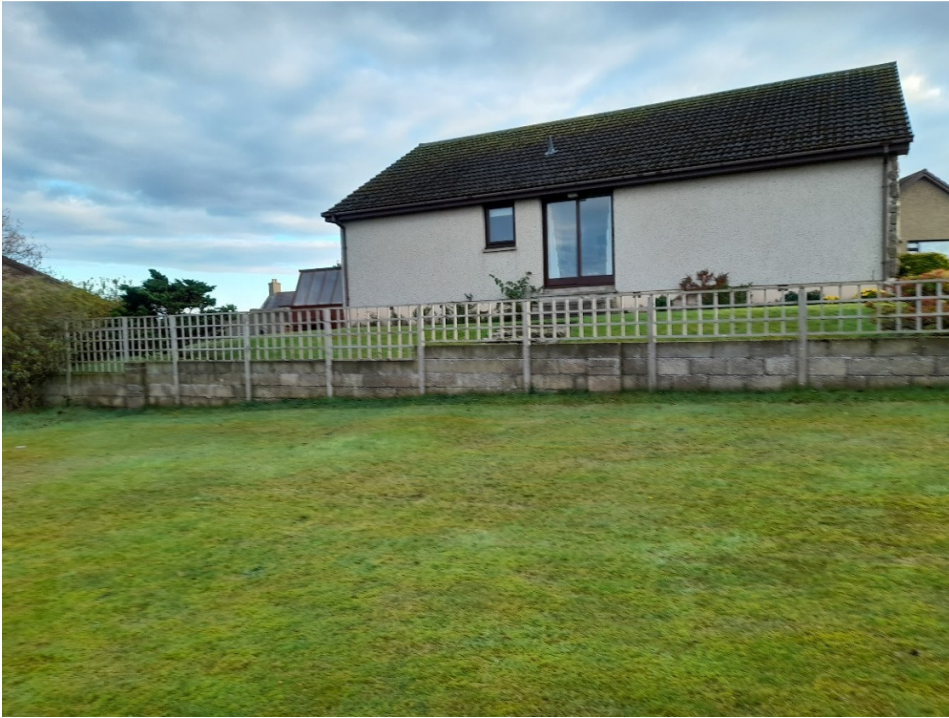
No 35 Adjacent to application site showing patio doors and change I level.
