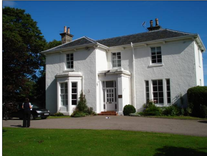
Photo 1 – Front elevation of the Old Manse
