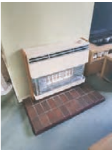
Old Baxi heating system with gas fire in living room
