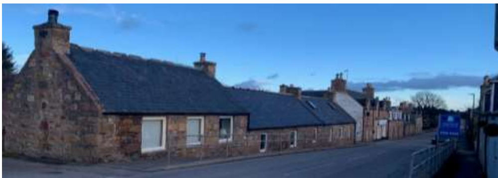
A row of properties (located on main road opposite hotel) with UPVC installations
