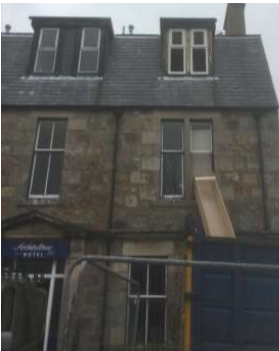
Hotel 1881 Before Window Replacement
