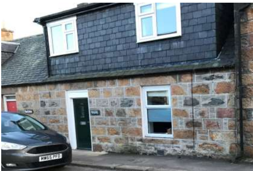
Another example of a property (located on the main road) with UPVC windows and door
