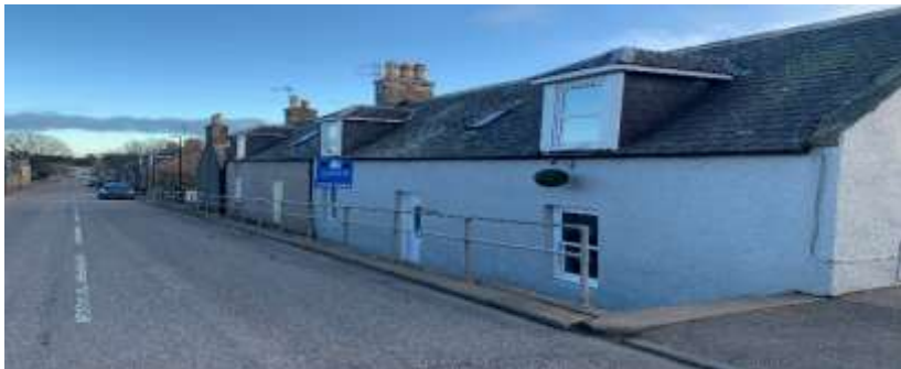
Another example of a property (located next door to hotel) with UPVC Upper Windows
