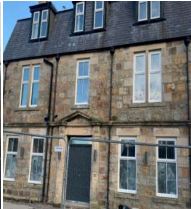
Hotel 1881 After Window Replacement
