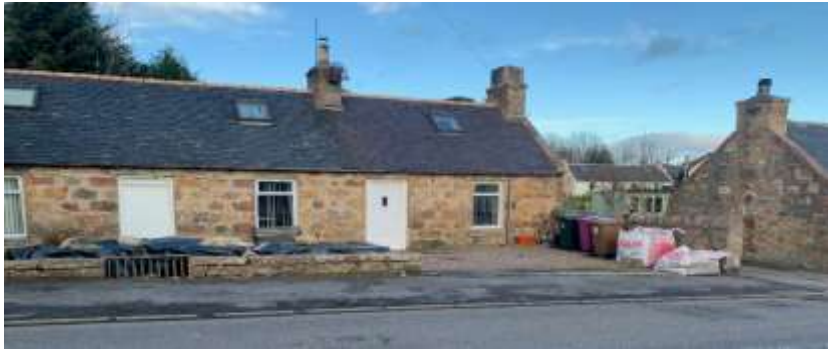
Another example of a property (located on main road) with new UPVC windows and door
