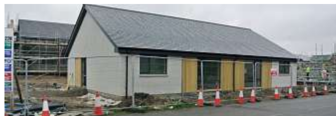
Progress being made on our new build homes in Hopeman
