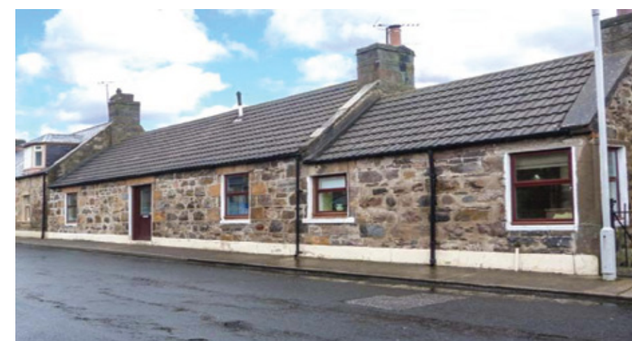
Typical planned village street in Moray
