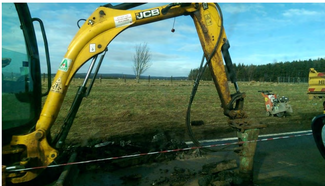
Photograph 3.6 – A95 Route Maintenance
