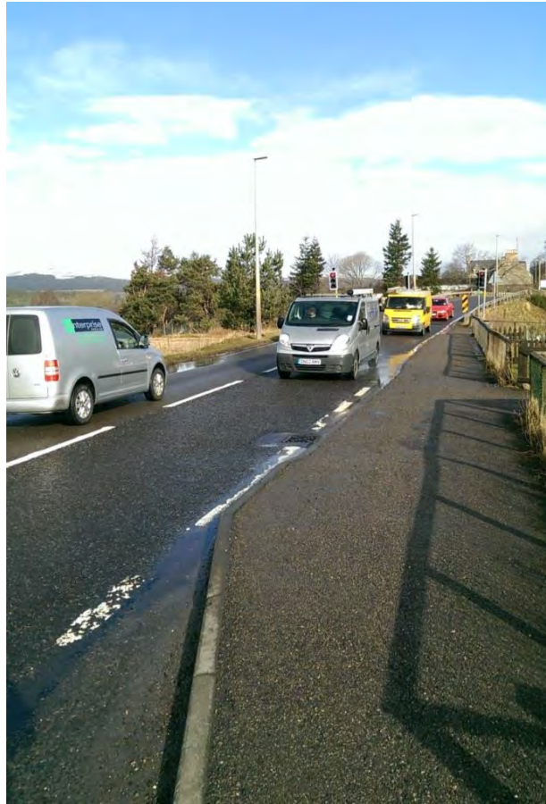
Photograph 3.3 – A95 Pinch Point at Cromdale
