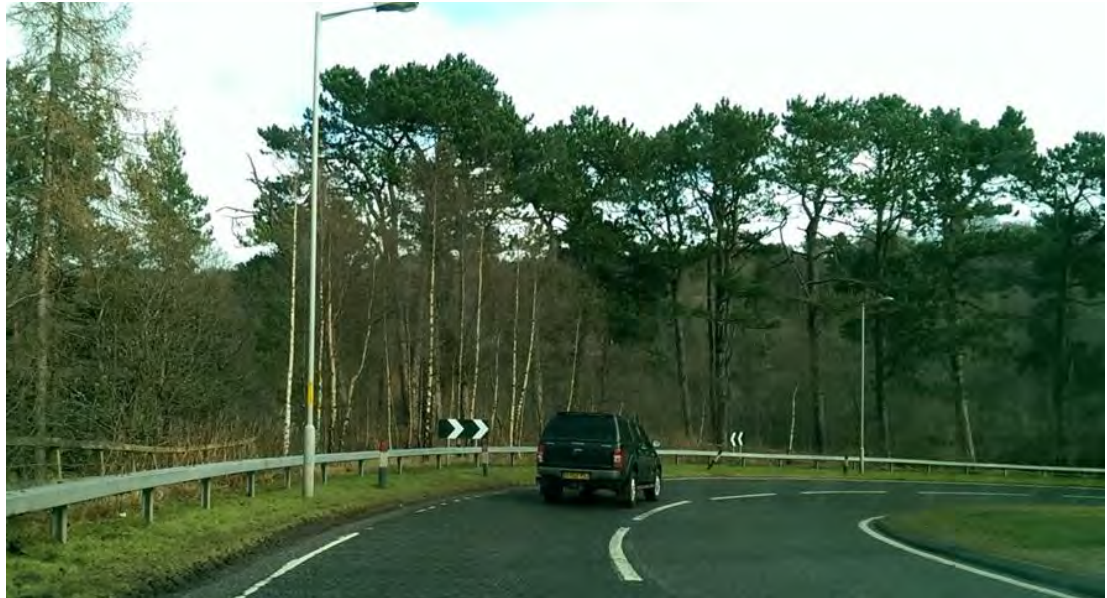
Photograph 3.3 – Example of significant horizontal change on the A95
