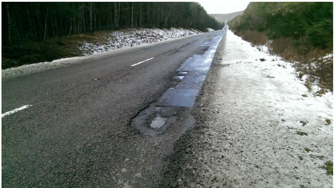
Photograph 3.5 – A95 Carriageway Breakup
