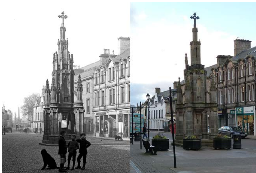
The historic photograph of the Market Cross c1875 reveals how much of the architectural detail of the monument has been removed during the constant repair programmes of the late twentieth century
