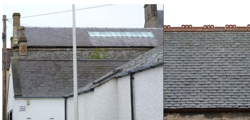
Varied roofscape in the left image, with a modern clay tile, sandstone and lead roll ridge; red clay cresting on the right
