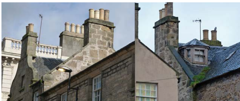
A key listed building on the High Street displays a lack of maintenance with a number of features failing: gutters need to be cleaned, roof slating needs to be overhauled, chimneyheads are leaning and bulging and have open masonry joints with missing stonework, and joinery needs decoration and repairs for which access is heavily constrained
