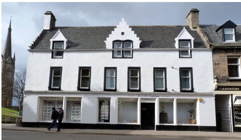
A range of Victorian cast iron shopfronts inserted at the ground floor of the earlier building at 117-121 High Street which carries the date of 1748
