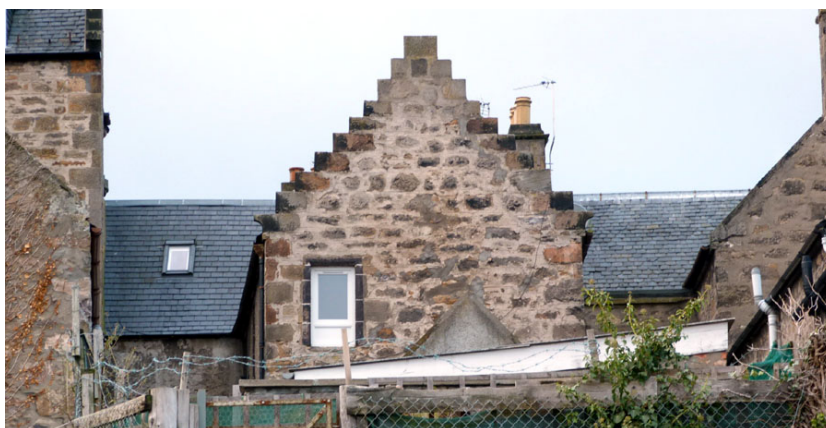
A wing to the rear of a listed building on the High Street displays a steeper roof pitch than would be the norm and crowsteps suggesting that parts of an earlier building could have been retained on the site: a chimneyhead at the gable has been taken down and the fabric modernised with modern windows and a new slate roof with a modern tile ridge
